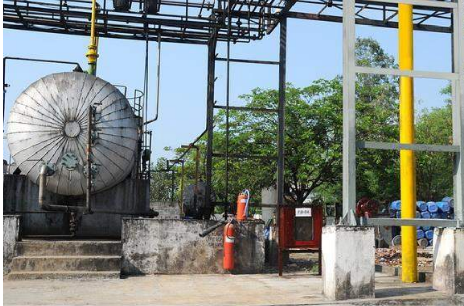
Fire Fighting Appliances Near Solvent Tank
